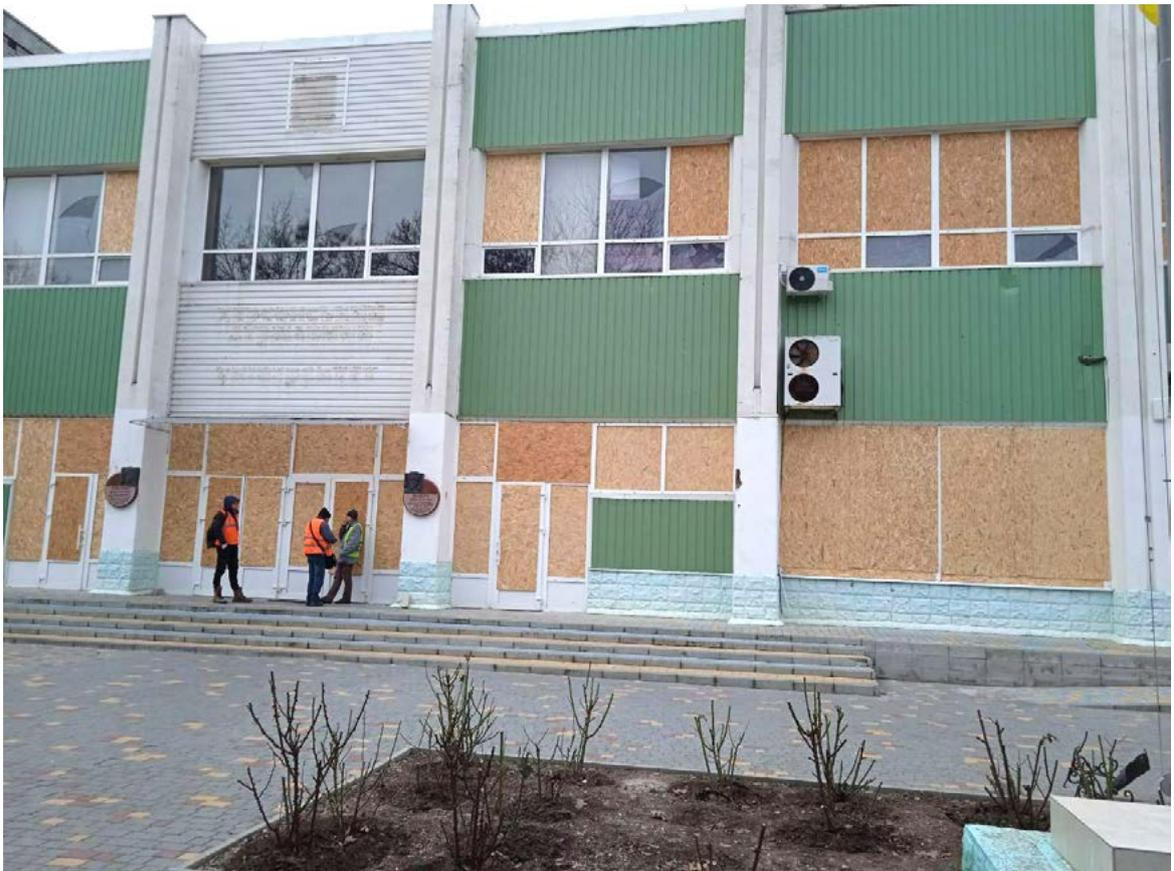
Bombing explosion waves damaged the façade and broke the windows of Kherson State University. After Kherson was deoccupied, the windows were temporarily “glazed” with OSB panels.
